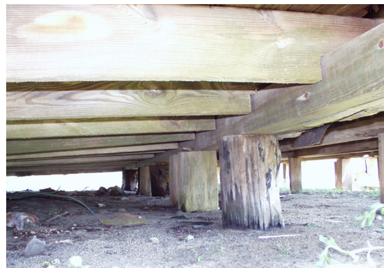
Figure 11 View northeast of front sill, showing typical joist/sill connections and wooden piers. (NPS-SERO-CRS, 2002)
