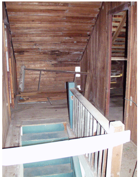
Figure 23 View west in second floor hall. (NPS-SERO-CRS, 2002)
