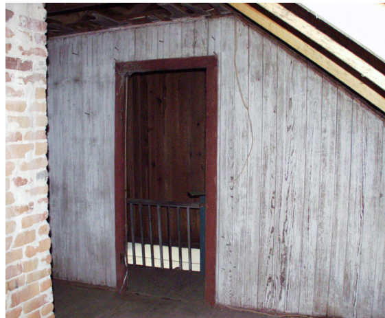
Figure 27 View south in Room 202. (NPS-SERO-CRS, 2002)
