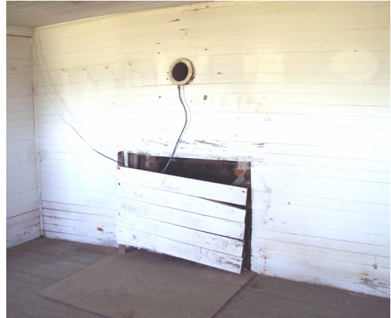
Figure 18 View of fireplace opening in Room 101. (NPS-SERO-CRS, 2001)
