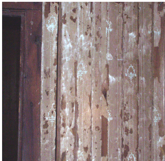
Figure 25 View of wallpaper-covered paneling on north wall of Room 201. (NPS-SERO-CRS, 2002)
